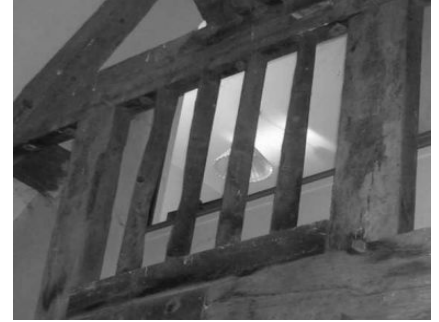
Mullion window (timber), with diamond mullions
